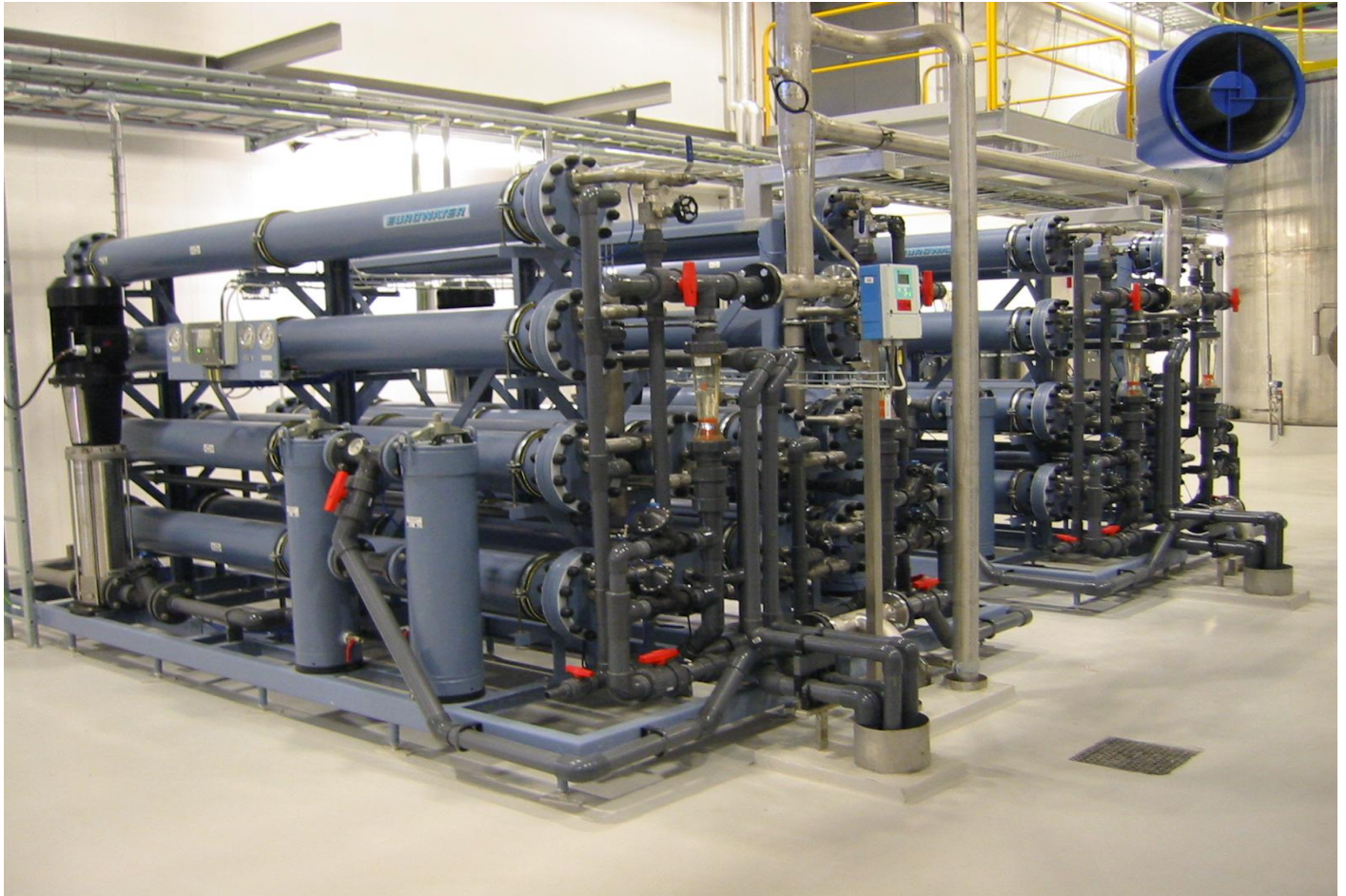
MediTec WP10S1MD brackish water treatment solution for 1.000.000 liters per day run on solar with battery backup.
